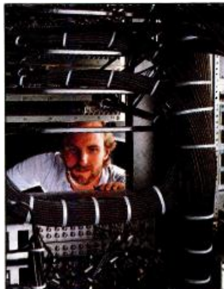
Neatly bundled and marked cables aid in troubleshooting and create a favorable impression on prospective clients.
